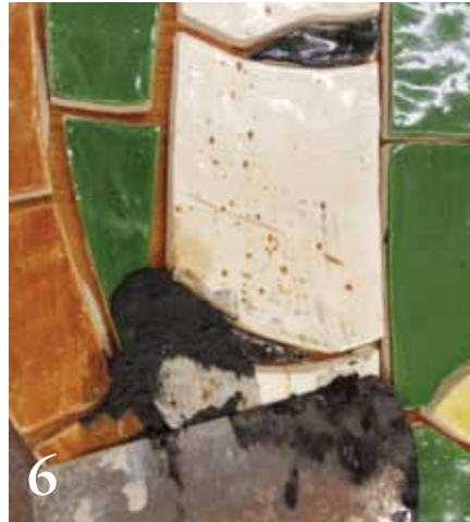
6 Pack the grout down between the tiles and spread it to fill each gap.
